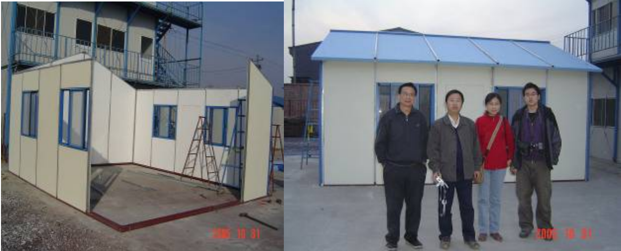
Fig.3 Erection of demonstration bamboo panel prefabricated house
