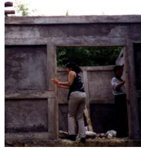
Fig. 1 water-containers and simple house being constructed of bamboo-woven concrete
