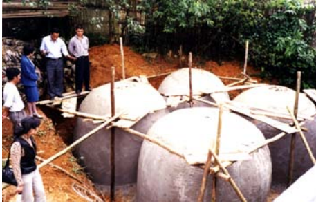
Fig. 1 water-containers and simple house being constructed of bamboo-woven concrete
