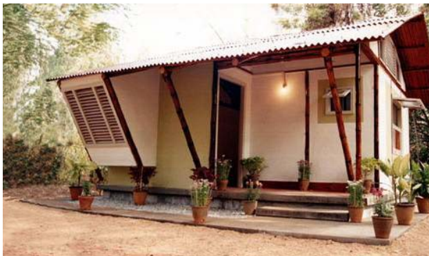
Demonstration House at IPIRTI – Bangalore, March, 2001
