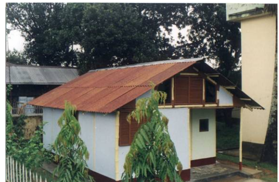
Bamboo House built at AGARTALA
