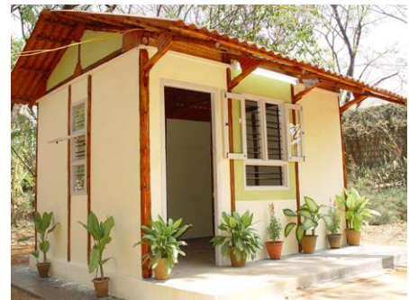
Security House at IPIRTI, Bangalore, 2004
