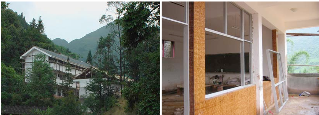
Fig. 4 + 5 Pingbian (Yunnan) school under construction.
