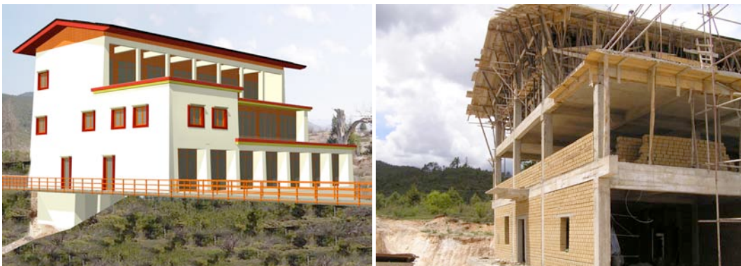
Fig 6 + 7 The EE-office in ShangriLa Botanical Garden under construction.
