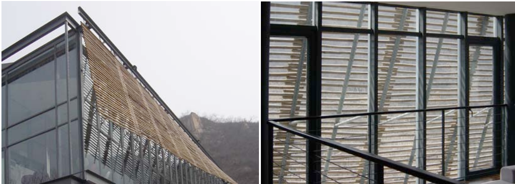
Fig. 2 + 3 A bamboo sunscreen that filters the incoming daylight at Badeling.
