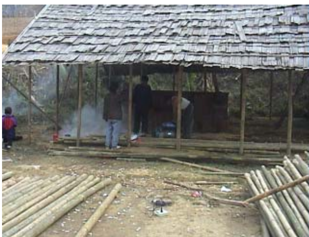
Preservation treatment facility
