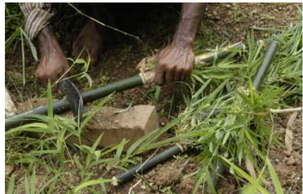
Cutting nodal sections from the culm
