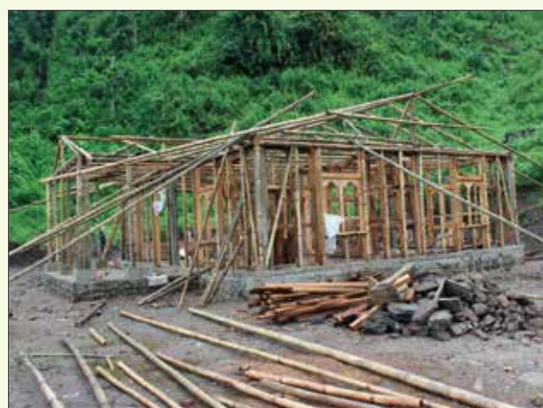
Figure 8: Bamboo/concrete frame hybrid under construction at Pakpay, Samtse
