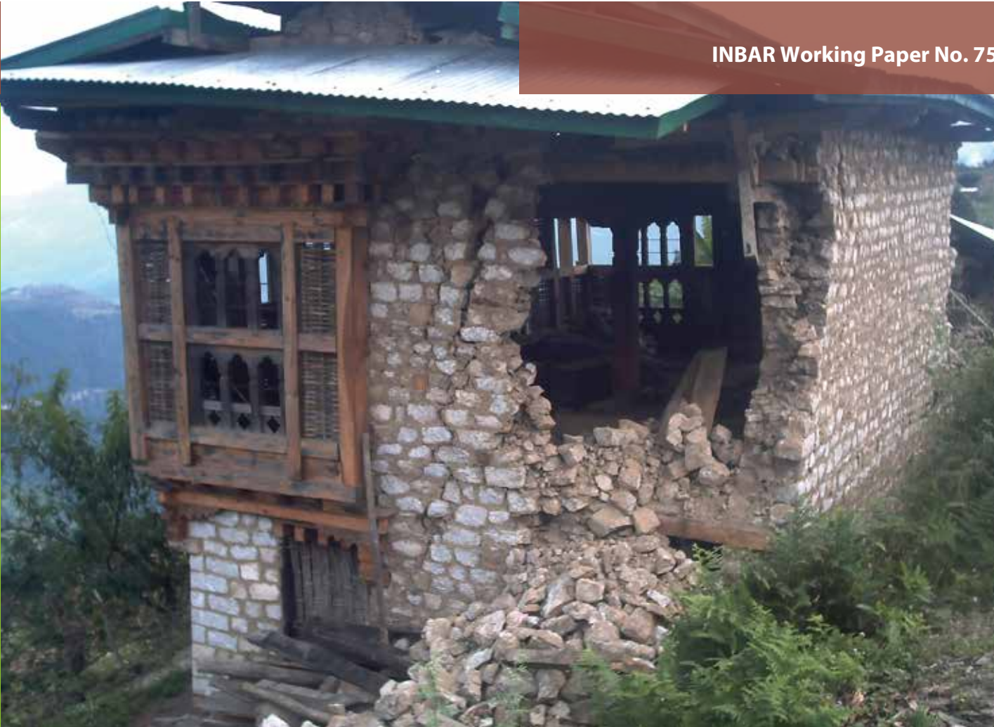
Figure 2: Damaged traditional timber & masonry structures after 2009 Mongar earthquake
