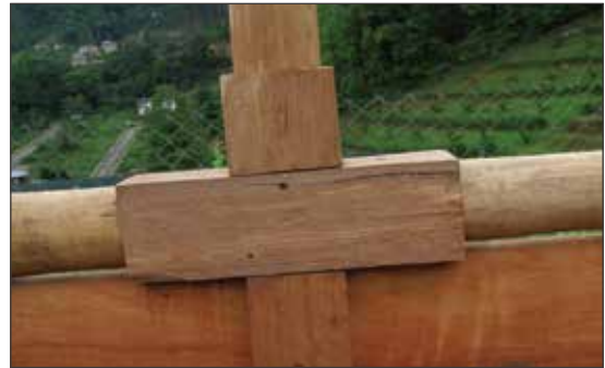
Figure 13: Bamboo-wood joint connecting two bamboo members
