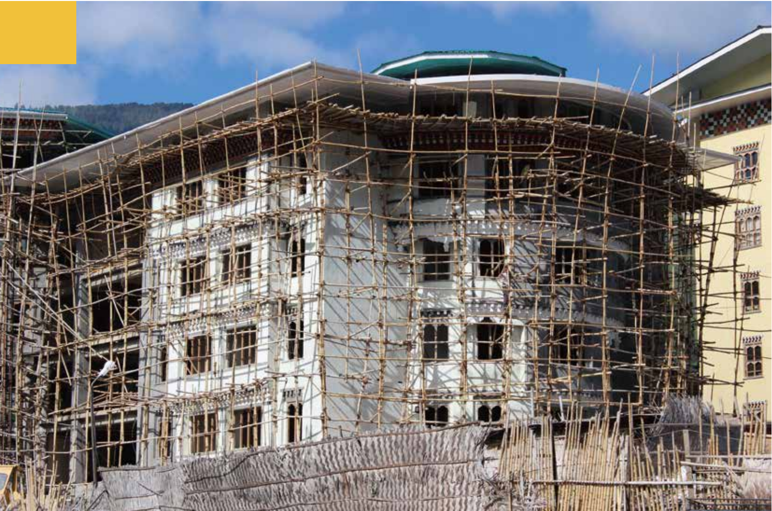
Figure 22: Bamboo scaffold in Thimphu, Bhutan
