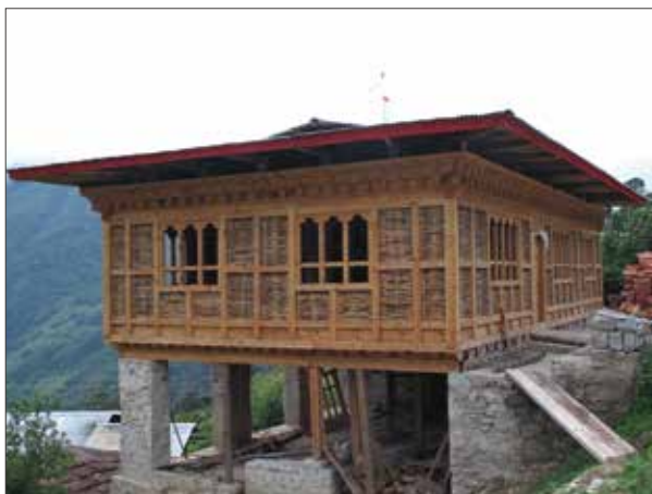
Figure 4: Traditional Bhutanese Timber Structure
