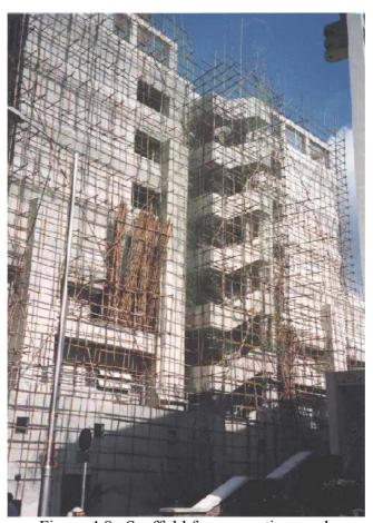
Figure 4.8 Scaffold for renovation work
