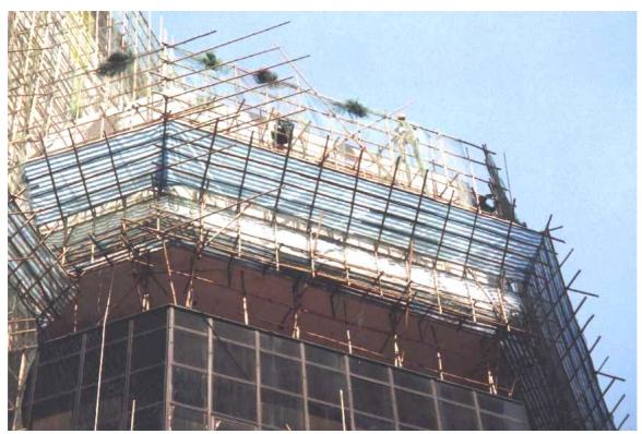
Figure 4.3 Catch fan in double layered scaffold
