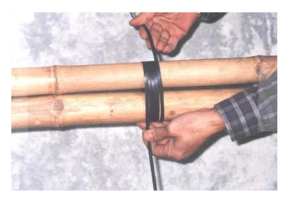
Figure 6.2 Tightening sequence of a lap in parallel members
