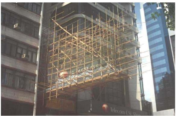
Figure 4.5 Cantilever scaffold for signage work
