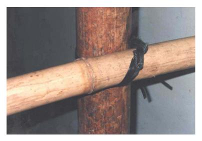
Figure 6.3 Tightening sequence of a joint between orthogonal members (continued)
