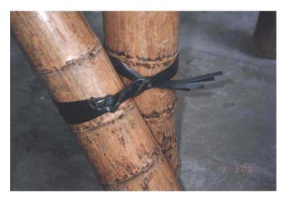
Figure 6.4 Tightening sequence of a restrained knot between inclined members
