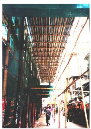
Figure 4.4 Obstruct plate in double layered scaffold
