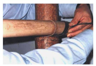
Figure 6.3 Tightening sequence of a joint between orthogonal members
