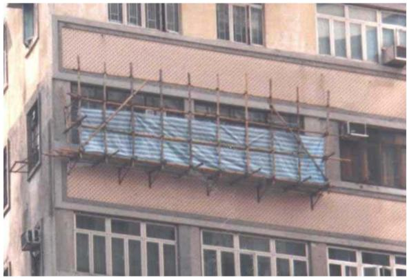
Figure 4.6 Truss-out scaffold for repair of external walls
