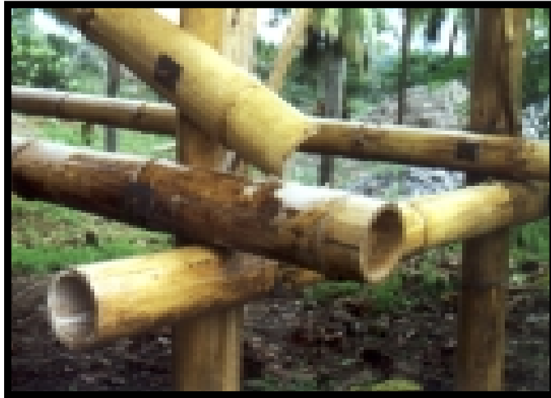
Fig. 64: A joint in Group 5, with steel bolts
