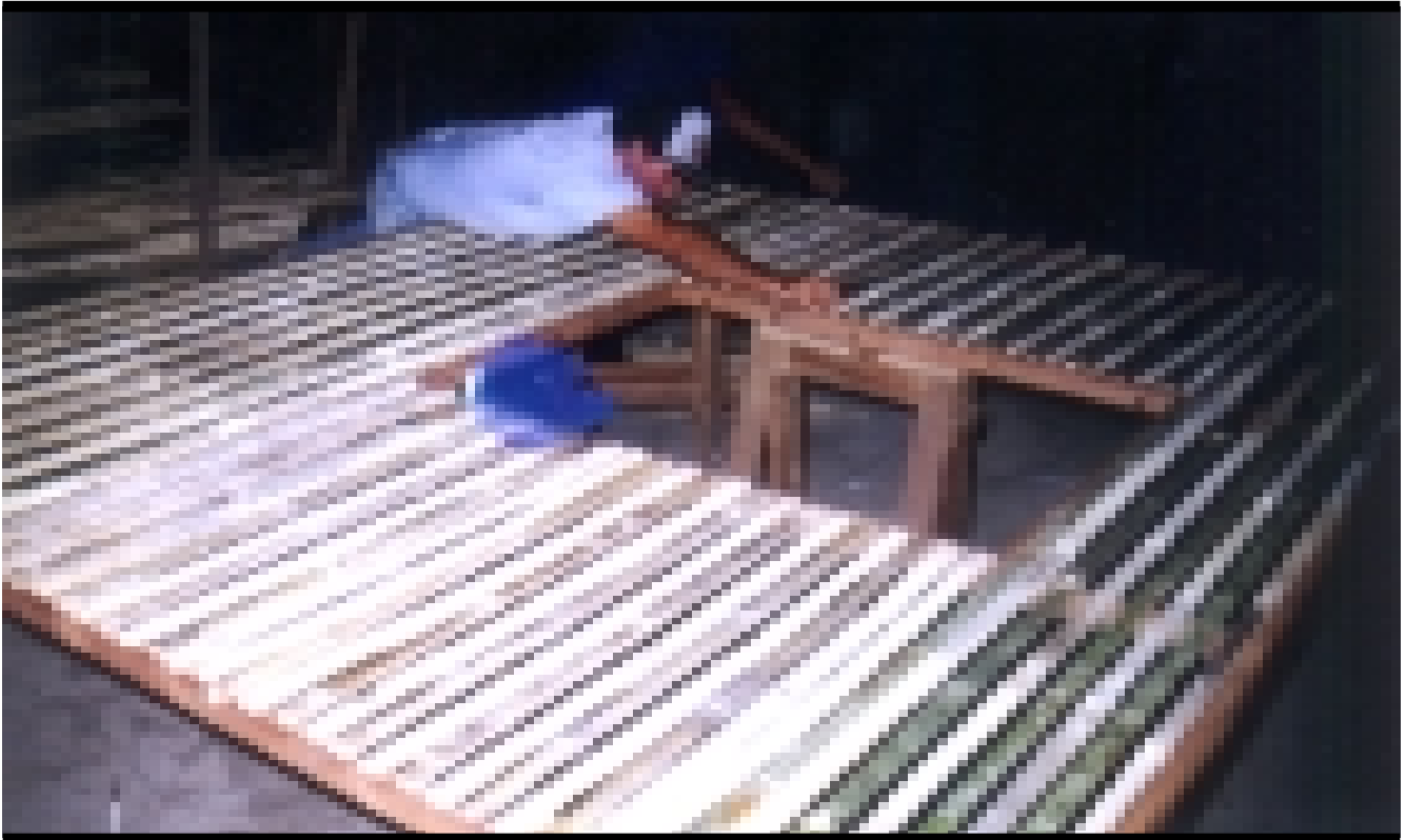
Fig. 19: Panels being prefabricated for mass housing
