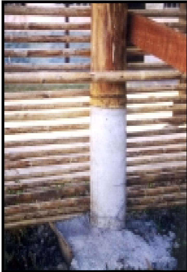
Fig. 18: Prefab concrete foundation for bamboo column
