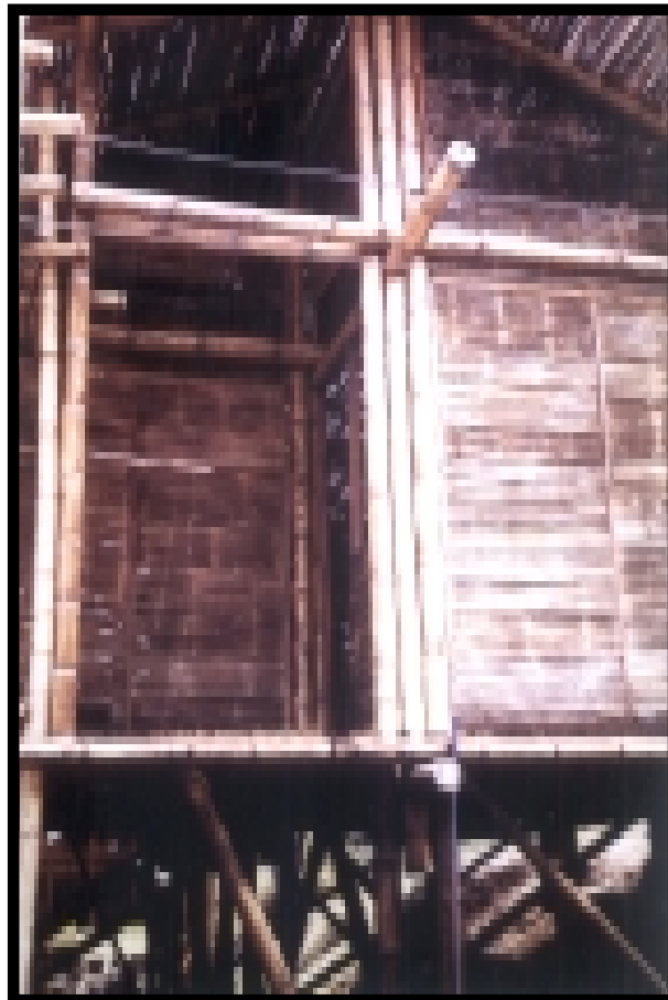
Fig. 94: A wall made of esterilla (Costa Rica)
