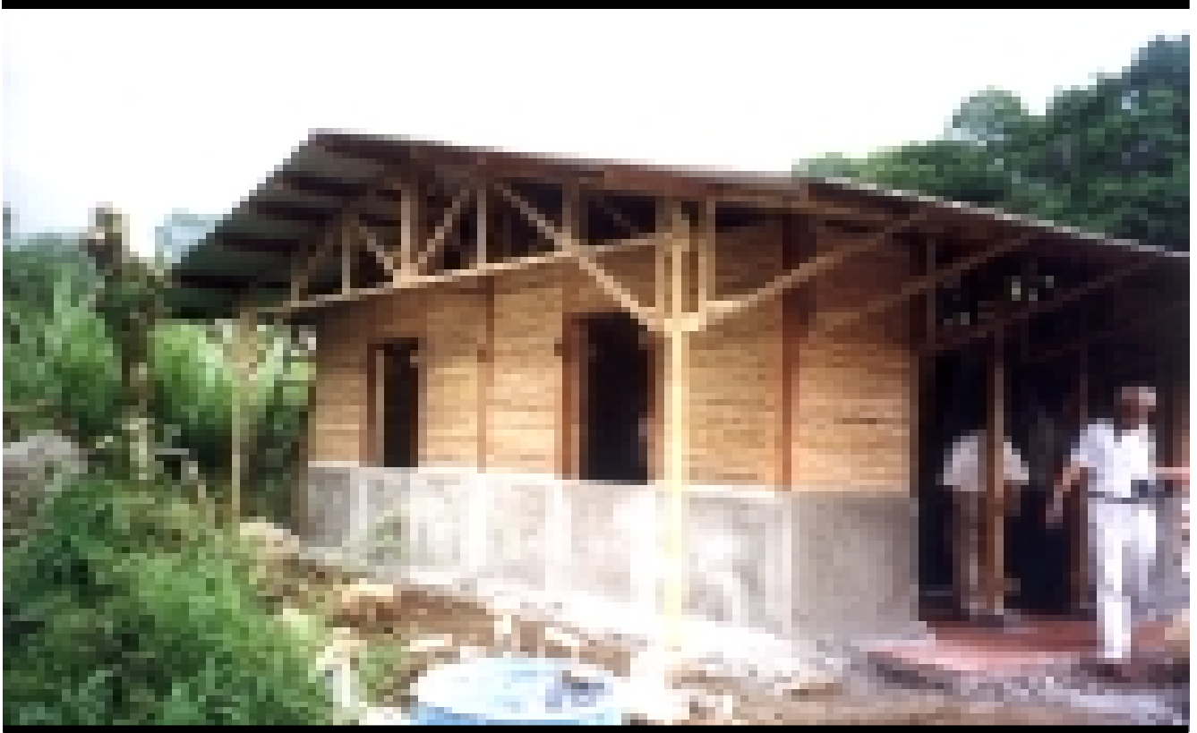
Fig. 92: A well-protected outside wall
