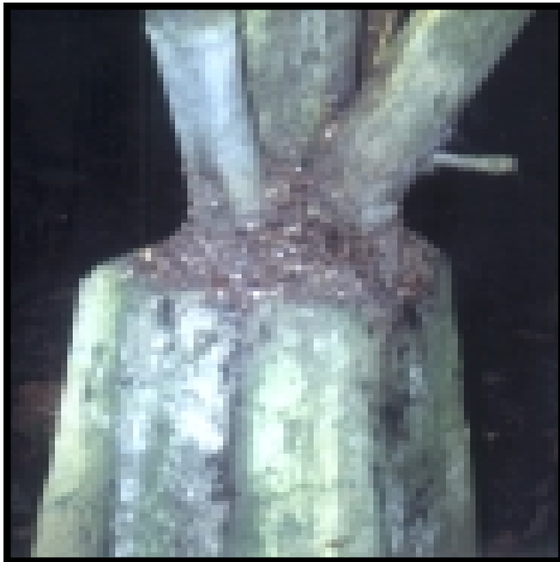
Fig. 36: Concrete foundation for a bamboo building, but the bamboo gets wet enough to invite fungal and insect attacks
