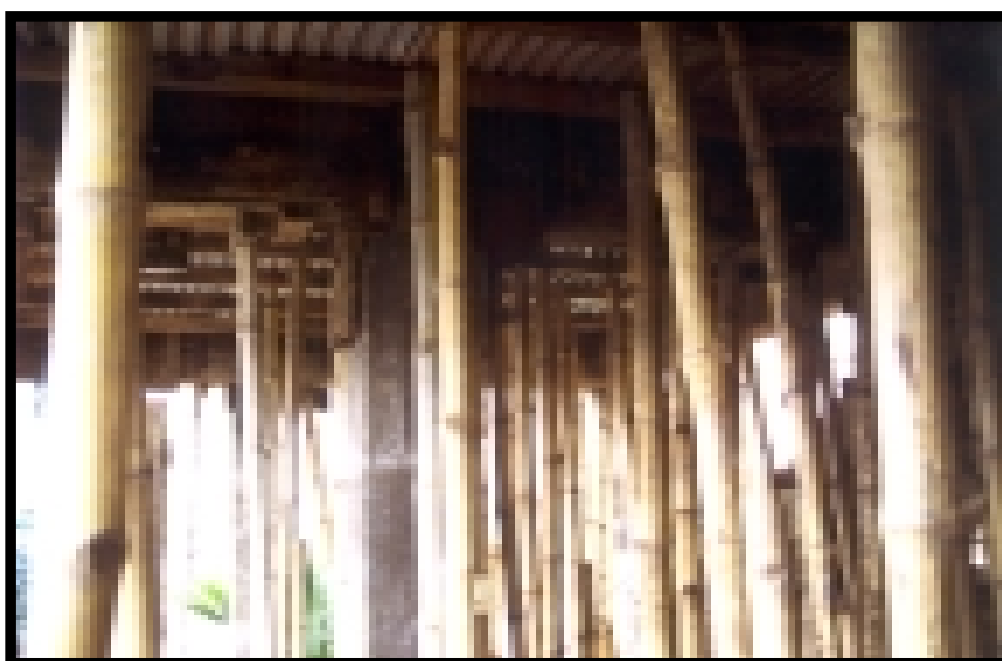
Fig. 84: Bamboo culms support concrete floor (Bangladesh)
