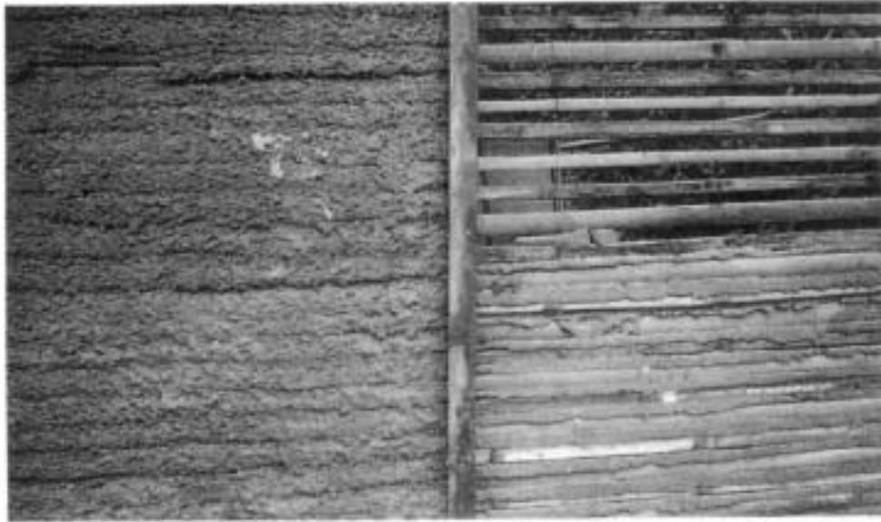
Fig. 18: Mounted paneling partially covered with cement/sand mixture
