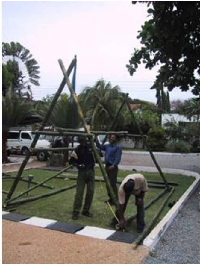
Picture 1: First two frames in place
