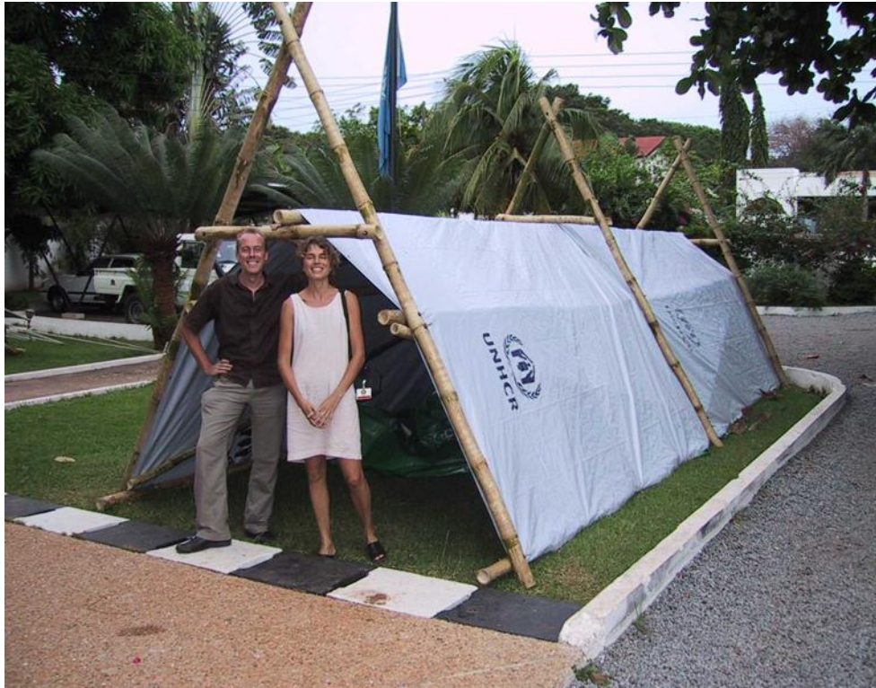
Picture 6: Second roof cover in place
