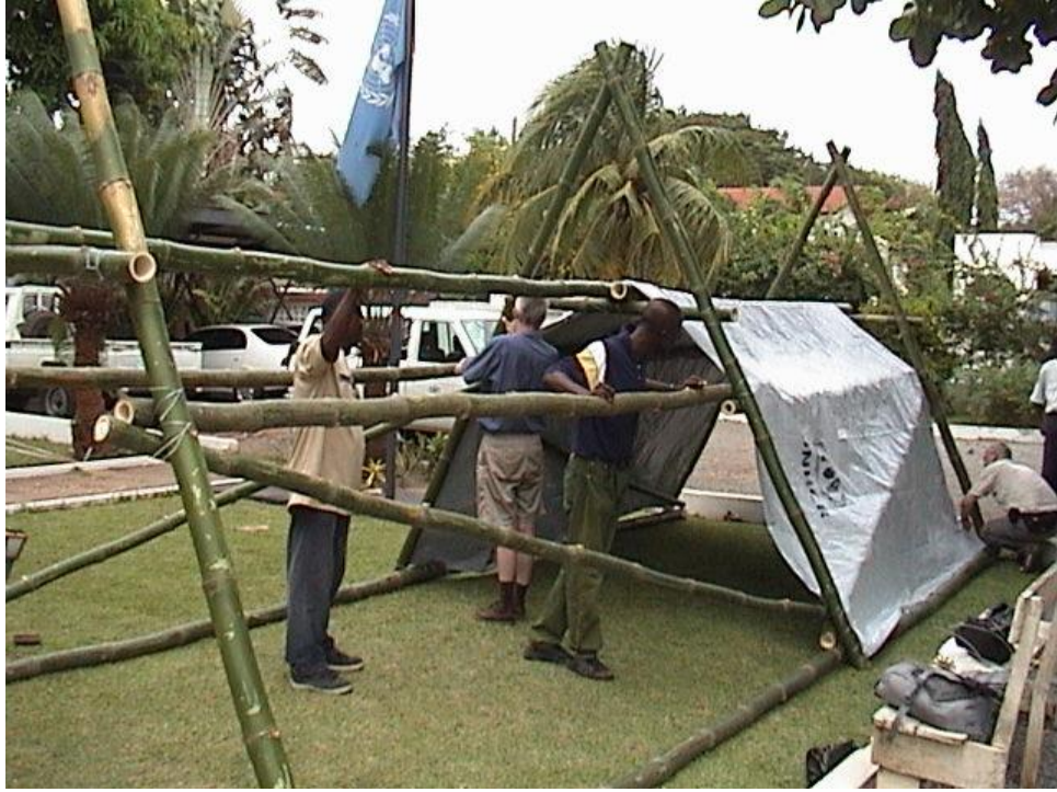
Picture 5: First roof cover in place
