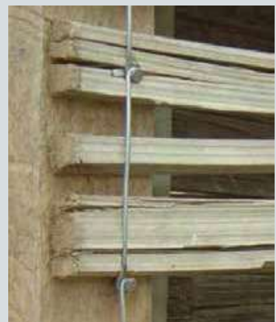
Final nailing after assembling the wire
