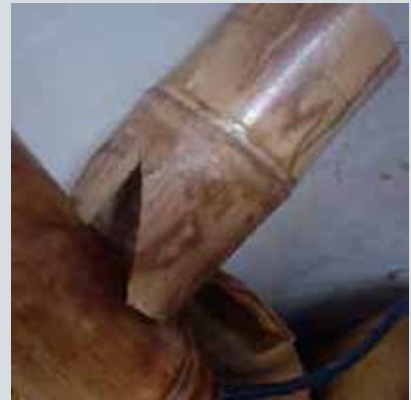
Application of a flute peak with a flange
