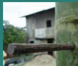
Wooden dowel embedded as anchor
