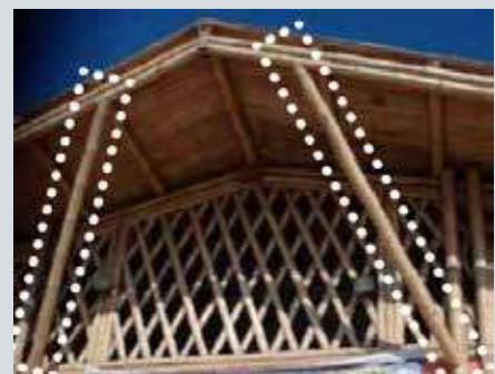
“Friend Foot” brace supporting the eaves.
