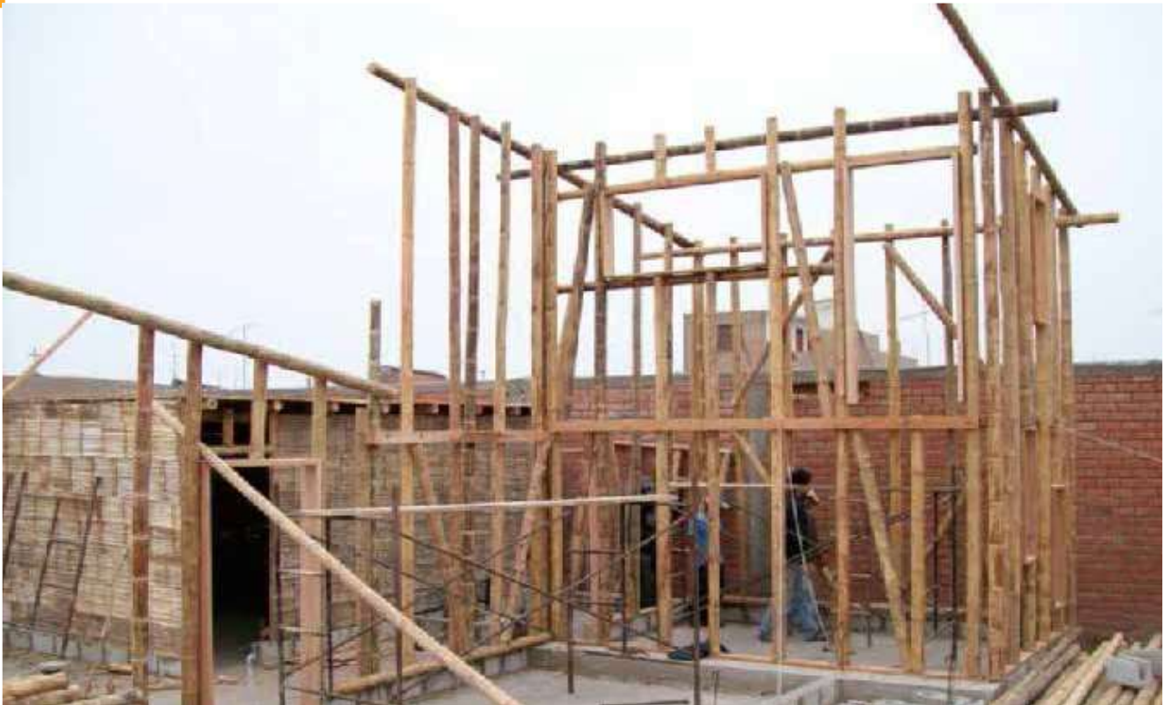
Constructing the bamboo structure over the foundation
