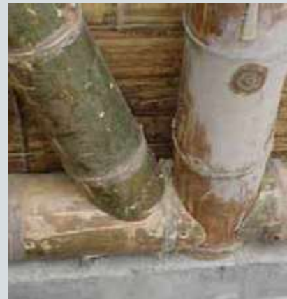
Application of a flute peak & a fish mouth cut
