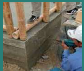
4 Pre-drilling with an extension bit
