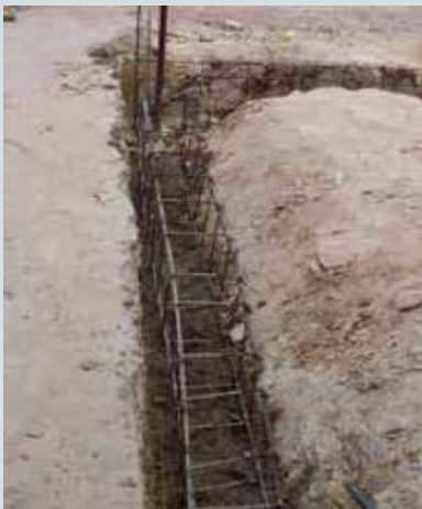
Foundation Excavation with Steel Reinforcement
