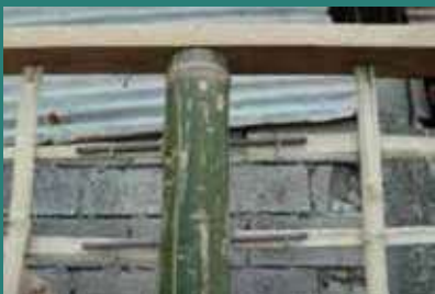
Tie rods or dowels passing through canes located in the middle of a wall.
