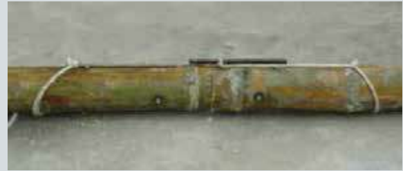
Two rods joined with pressure rope and placement of two bolts.
