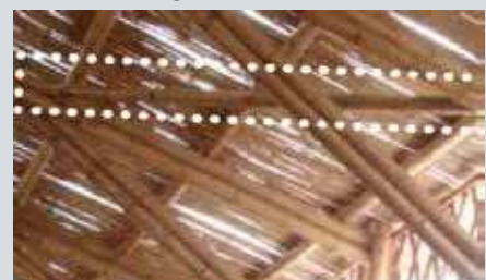
Collar ties ensure the rigidity of the roof.
