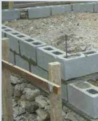
Foundation Wall over Foun- dation Base
