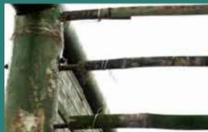
Single-side anchors in vertical canes at the end of the wall.
