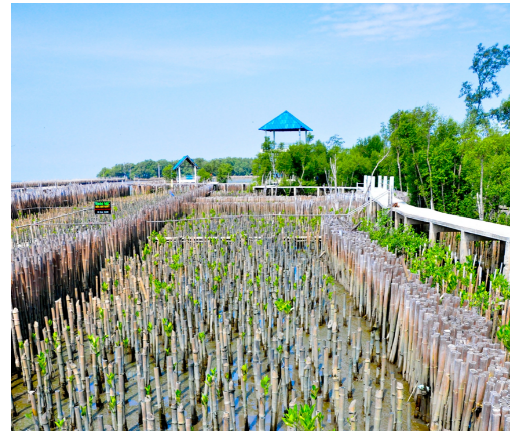
Figure 29. Bamboo dam and mangrove farm (source: somkku9kanokwan).
