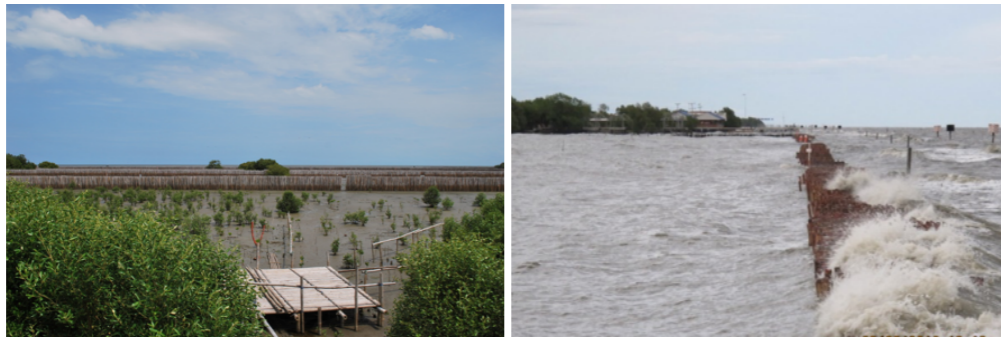
Figure 31. Assessments demonstrated that wave heights declined significantly behind the bamboo walls constructed at Pak Klong Bang Bo. (source: Bamboo Revetment Project) (DCMR, 2014).
