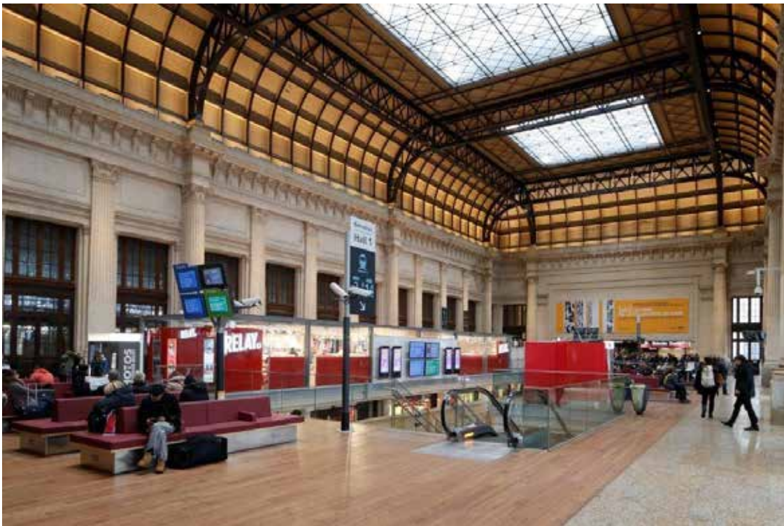
Figure 2: Ultra density SWB flooring in Bordeaux train station, France. This was used due to its hardness and wear resistance. (Photo credit: MOSO International)
