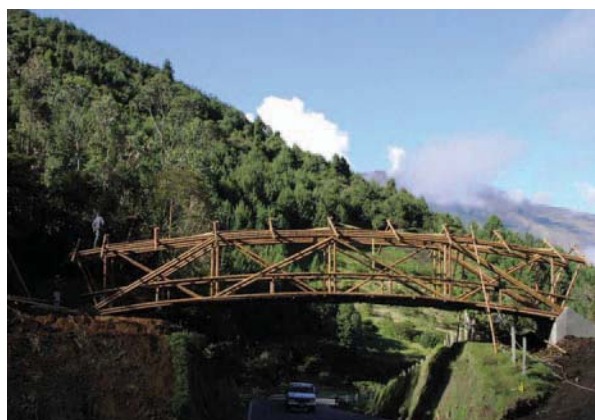
German architect Jorg Stamm has successfully implemented several construction projects in Colombia. Among them is a bamboo bridge with a span of 52 m.
