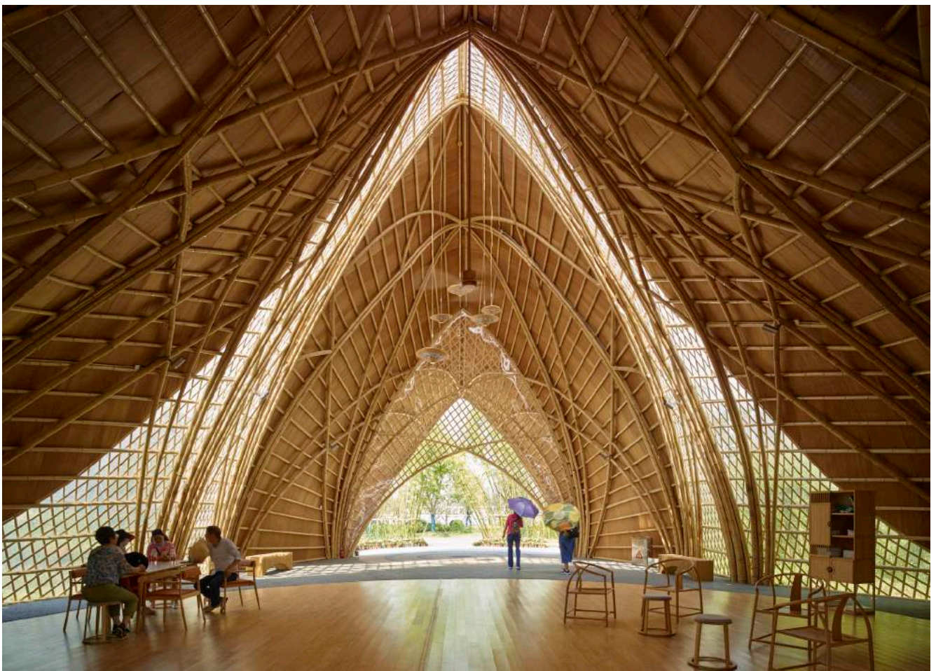
The Fish-shaped Bamboo Pavilion, located in the north of the INBAR Garden, was a 280-square-metre structure made using round bamboo. From above, the Pavilion resembled the shape of a fish: an auspicious symbol in Chinese culture. The Pavilion shows how traditional bamboo building materials can be used to create modern architectural structures.
